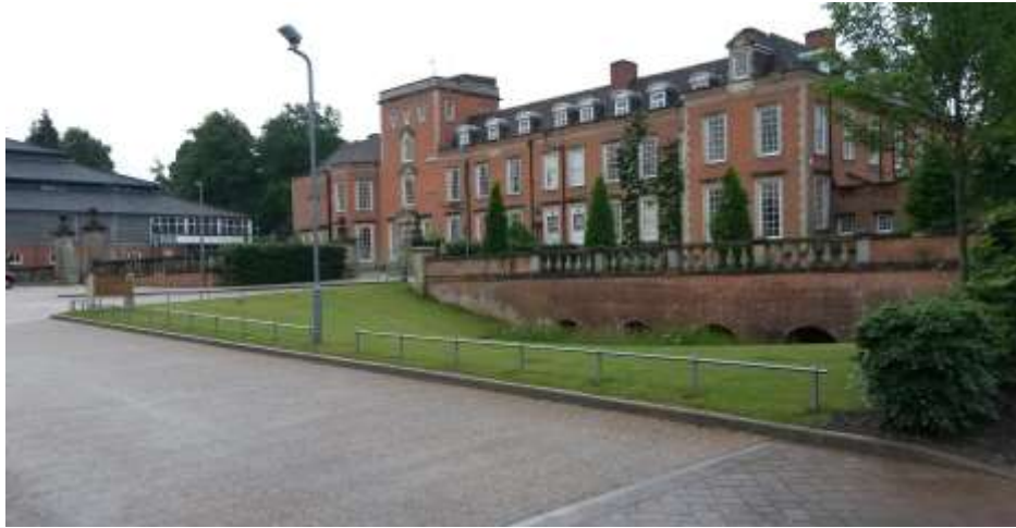
South Hill Park Mansion (Wilde Theatre on left)
