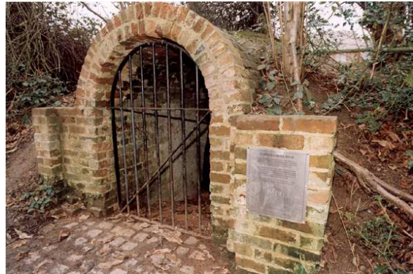
Plate 2 An Icehouse (grade II Listed Building)
