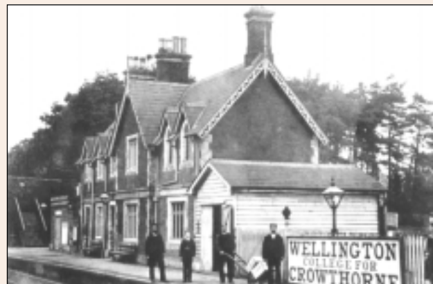
Wellington College Station, Crowthorne in C.1895
