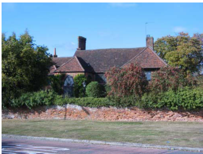
Eroded brickwork in the listed wall at Binfield Place
