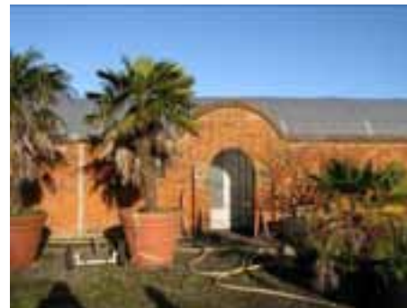
One of the repaired brick entrances into the Walled Garden
