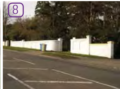
8 Characteristic boundary treatment along London Road
