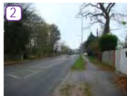
2 Western section of London Road is of lesser quality
