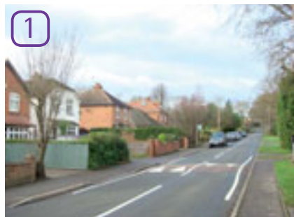
1 Detached houses alongside Wellington Road
