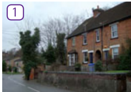
Retaining wall creates distinct boundary treatment
