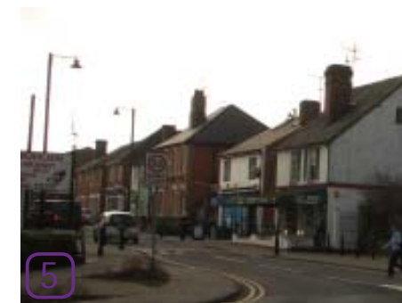
5 Victorian houses on Lynch Gate
