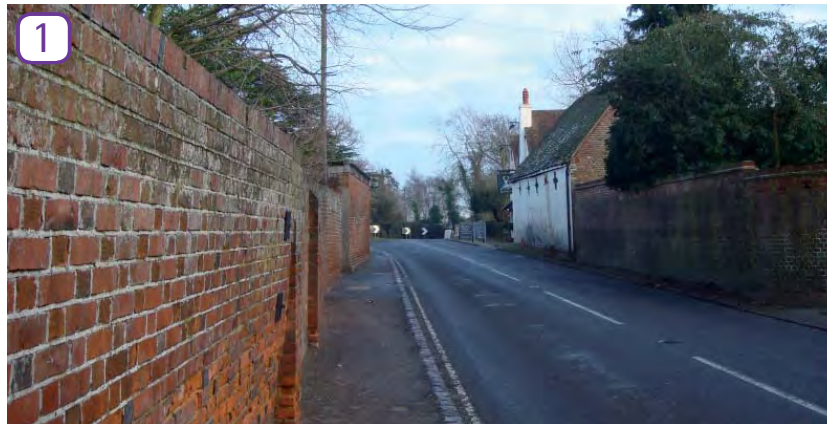
1 Approach into Winkfield from the west is defined by high degree of enclosure and distinct character of walls.
