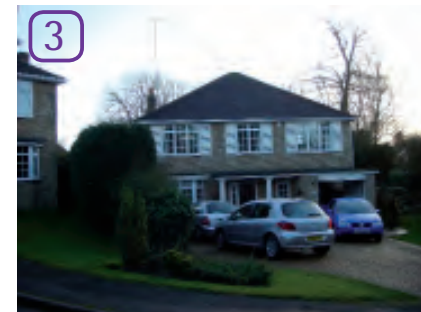
3 Development at the bottom of Pump Lane does not contribute to the overall character of this area or that of Cheapside as a whole.
