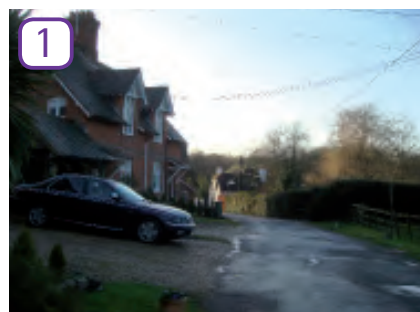
1 Cottages fronting onto Pump Lane
