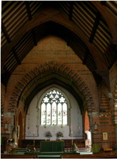
Plate 41: The interior of the Church with Blomfield's distinctive design and Kempes east window
