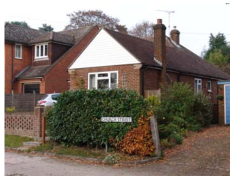
Plate 36: New buildings should try to harmonise, by matching the existing hierarchy of height and space
