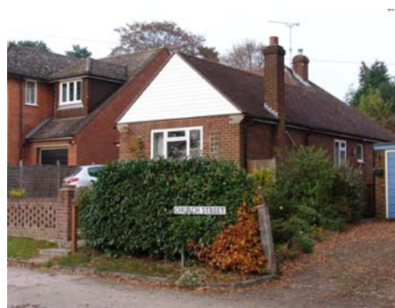
Plate 20: No. 55 Church Street
