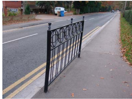
Plate 32: The pedestrian barrier along Waterloo Road using traditional ironmongery
