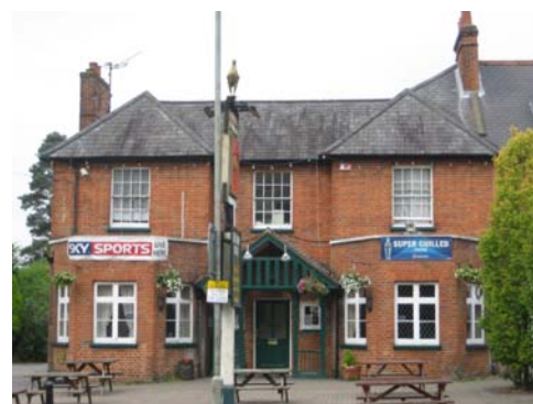
Plate 30: The Iron Duke Public House
