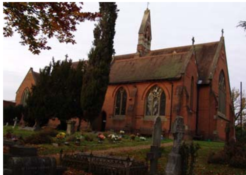
Plate 11: The architectural and historic character of the St. John the Baptist's Church is central to the area (Southern elevation)
