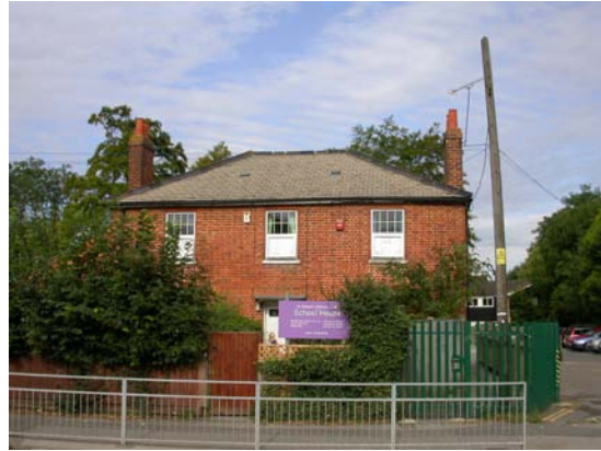
26 St Michael and Mary's Church school, Rectory Lane, looking west
