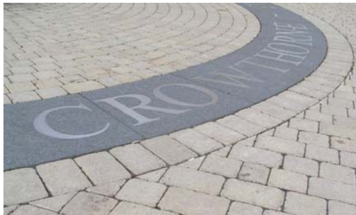
Photo 1 – Paving at Crowthorne Square
