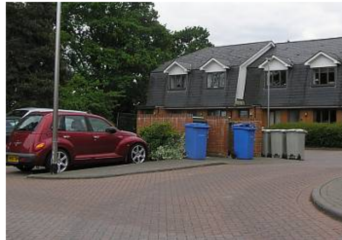
The above bin storage area is visually dominant and poorly screens bins within the streetscene
