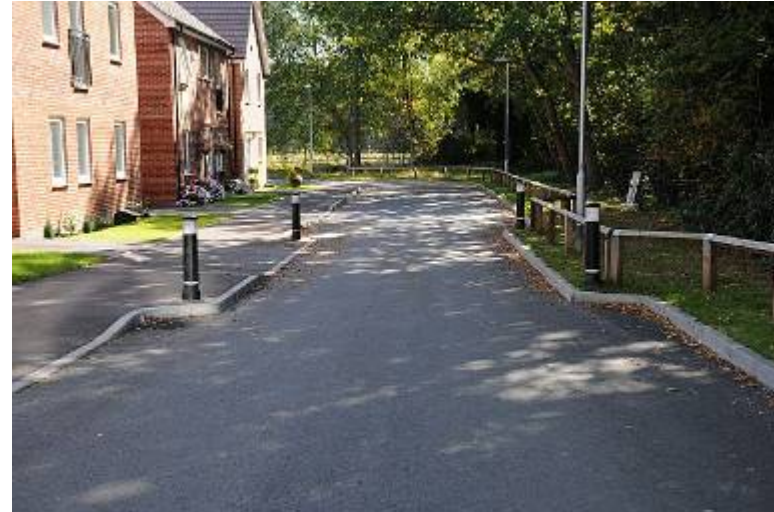
Acute angles of traffic calming design makes street cleansing difficult
