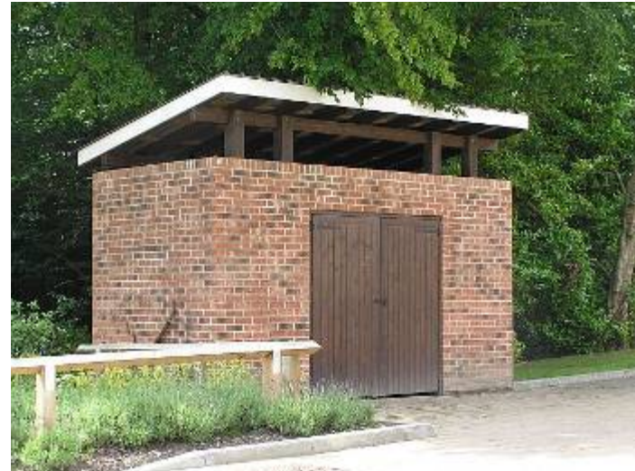
Bin store designed in keeping with apartment block at The Parks development in Bracknell. The brick matches the buildings, the roof follows the asymmetric design seen throughout the development and an area of planting provides a buffer within the streetscene
