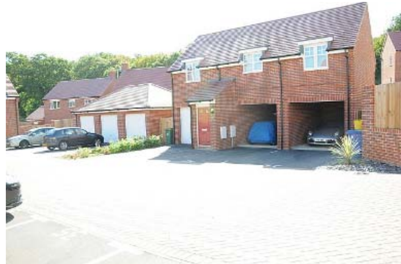
Car ports in use, however, the garages have cars parked to the front
