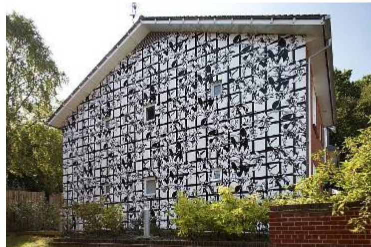
Richard Woods at Mabley Court, Easthampstead, Bracknell
