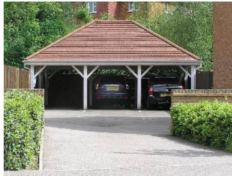
Car barns being used for parking
