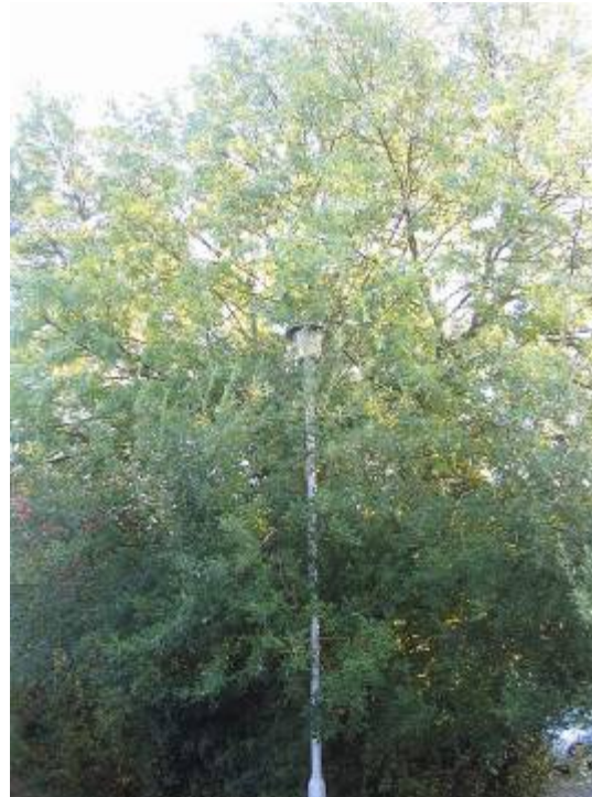
Street lights and trees in conflict
