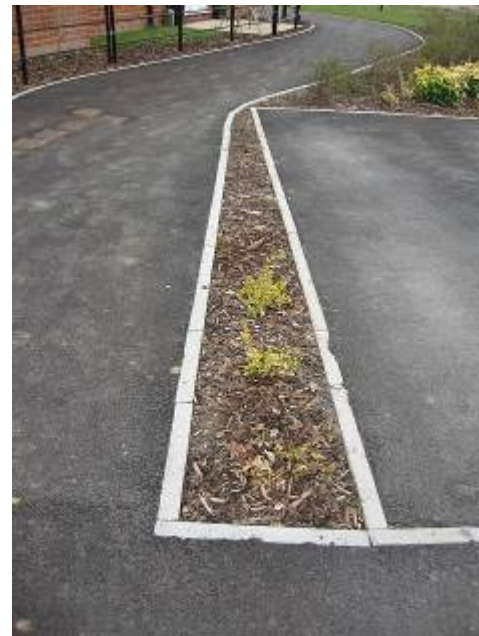
This planting strip is too narrow to support any planting of substance
