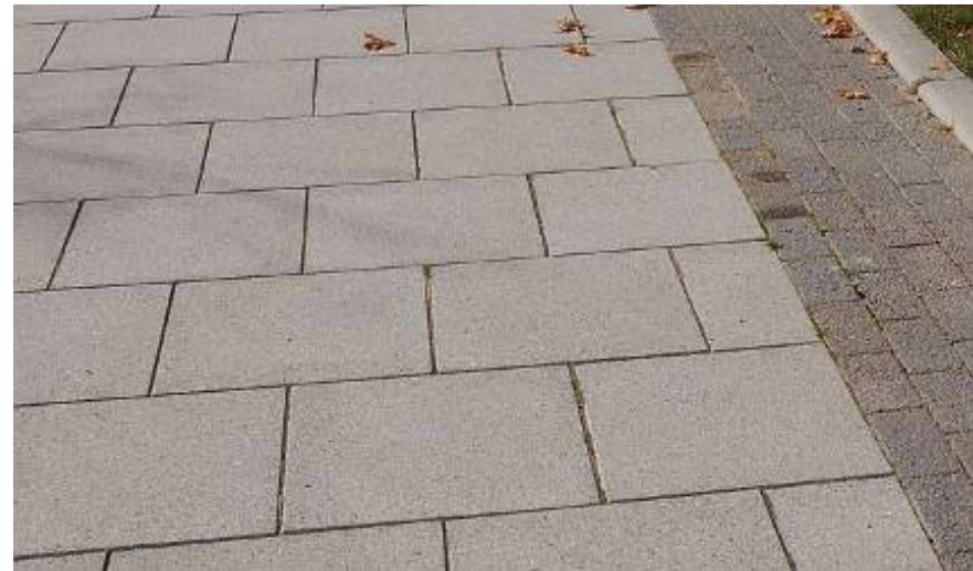
Concrete slabs used on a pavement in a Feature Square at Jennett's Park
