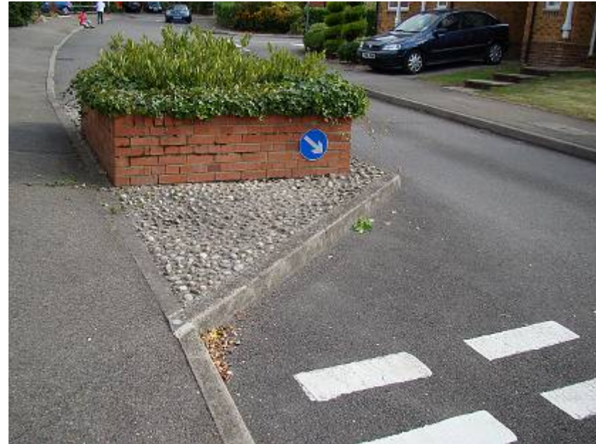
Planters used as a traffic calming method, however, traffic signs are unnecessary in such a low trafficked area.
