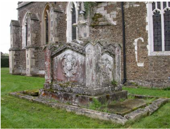
15 Stone tomb on north side of church, looking south-east
