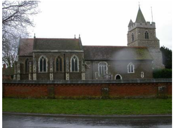
8 St. Michael's Church, looking south-east
