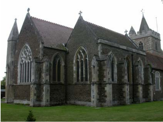
9 Gate and lane on west side of church, looking south-east
