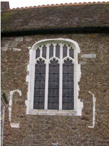
11 Blocked windows on north side of church
