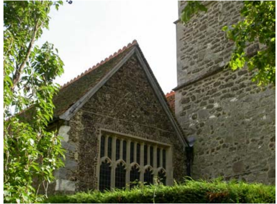
10 Roof scar on west face of north nave
