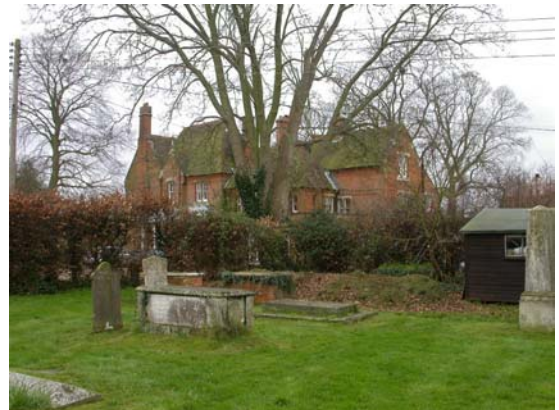
18 Herbert House, looking south-east
