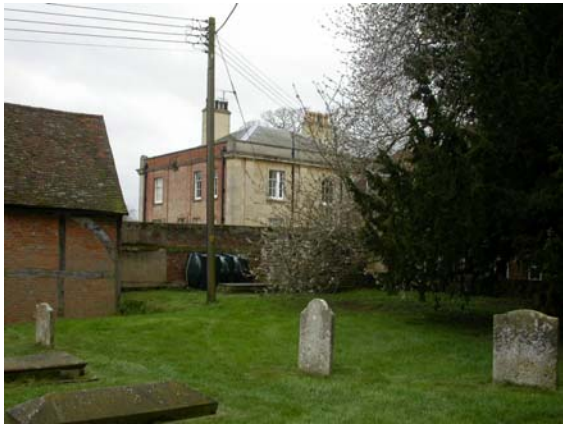
3 North and east sides of Rectory House from the churchyard.
