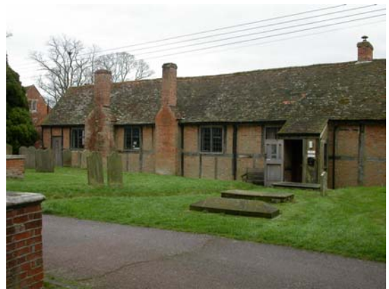
16 Church offices, south of the church, looking south
