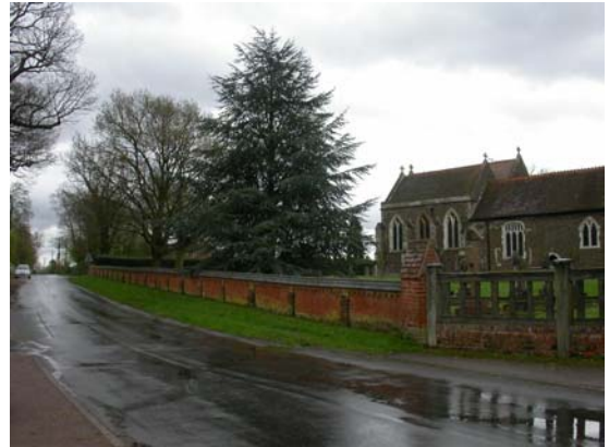
14 Boundary wall of church, looking east
