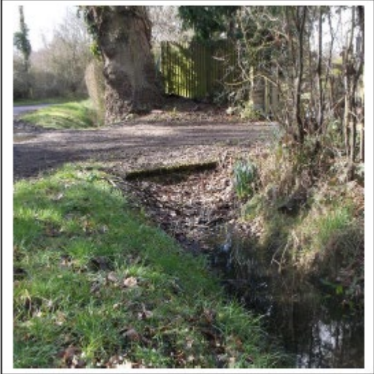
Figure 3 shows a ditch running between the public highway and a private estate which passes under an access way. The Riparian Owner of this ditch and culvert (a culvert is a length of ditch which has been piped) is the owner of the property next to the ditch. If the driveway gives access to more than one property, the Riparian Owner may wish to approach them to assist with the maintenance of the culvert.
