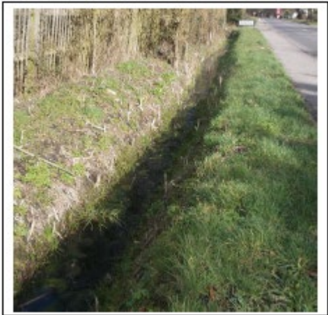
Figure 2: A ditch running alongside the public highway which is the responsibility of the private land owner.
