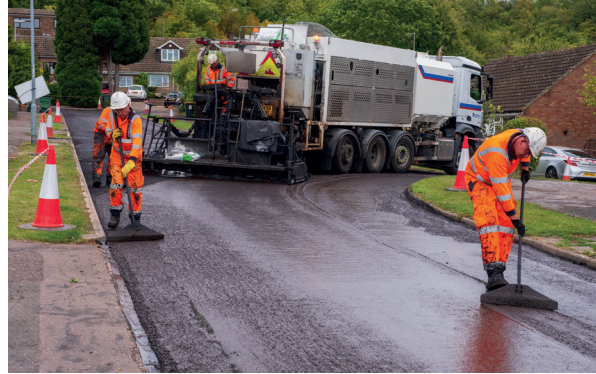
Micro-surfacing being applied to a road
