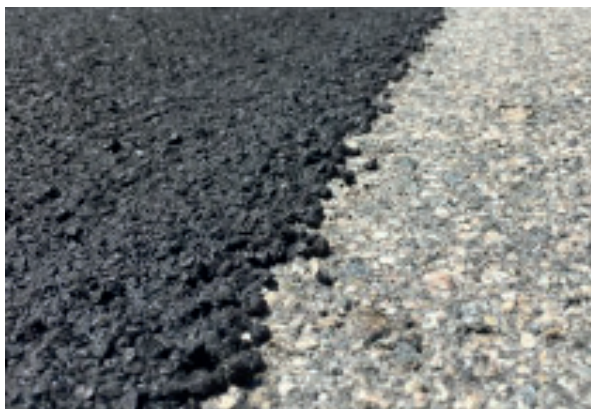
New micro asphalt surface (left side)
