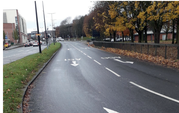
Completed micro-surfacing after 3 months once the material has bedded in and been swept.
