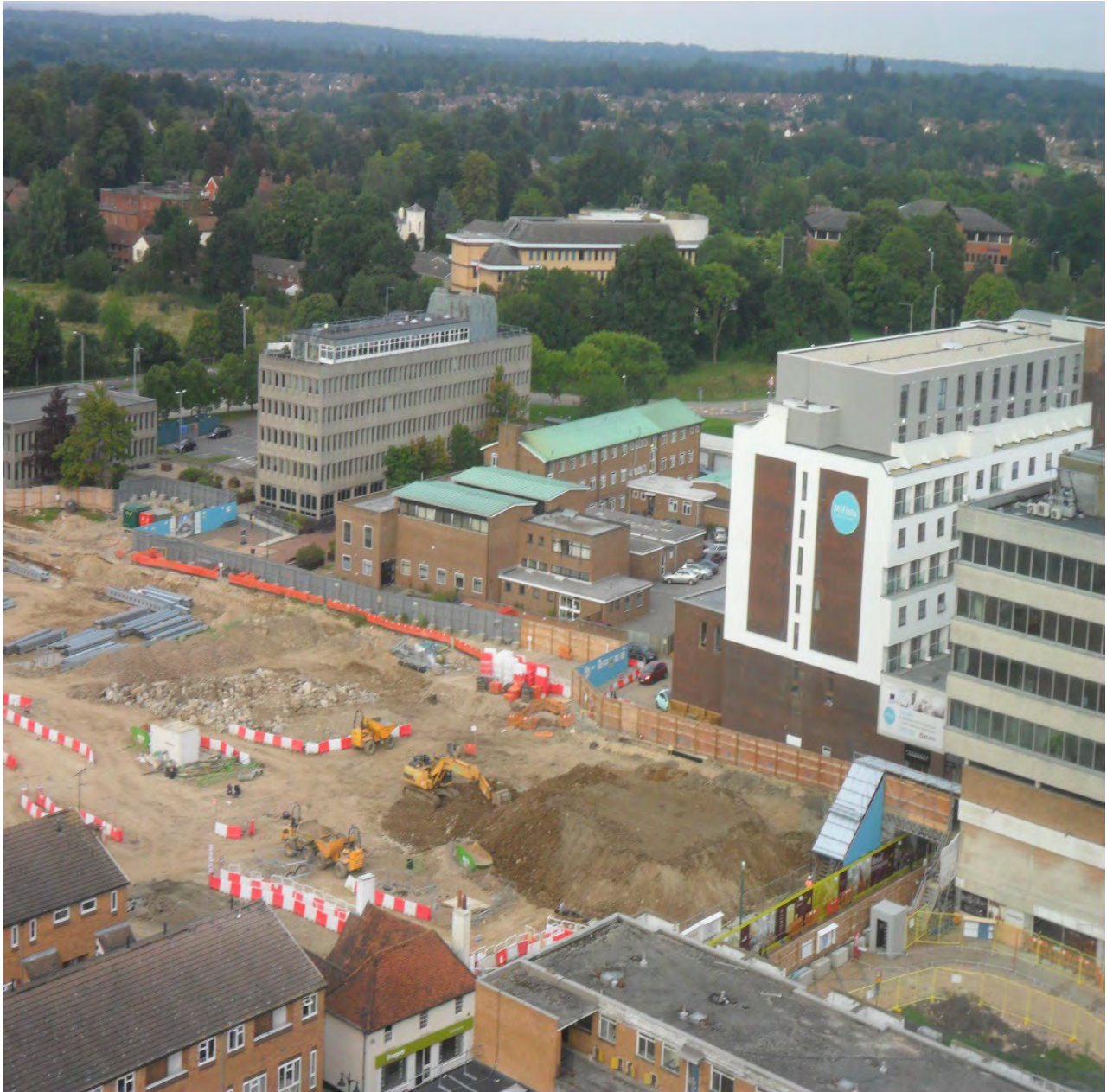
Illustration 1 Bracknell's new town centre retail regeneration takes shape, view from Ocean House, September 2015
