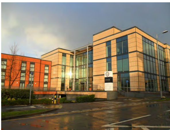
PW7: Origin Building, Western Road
