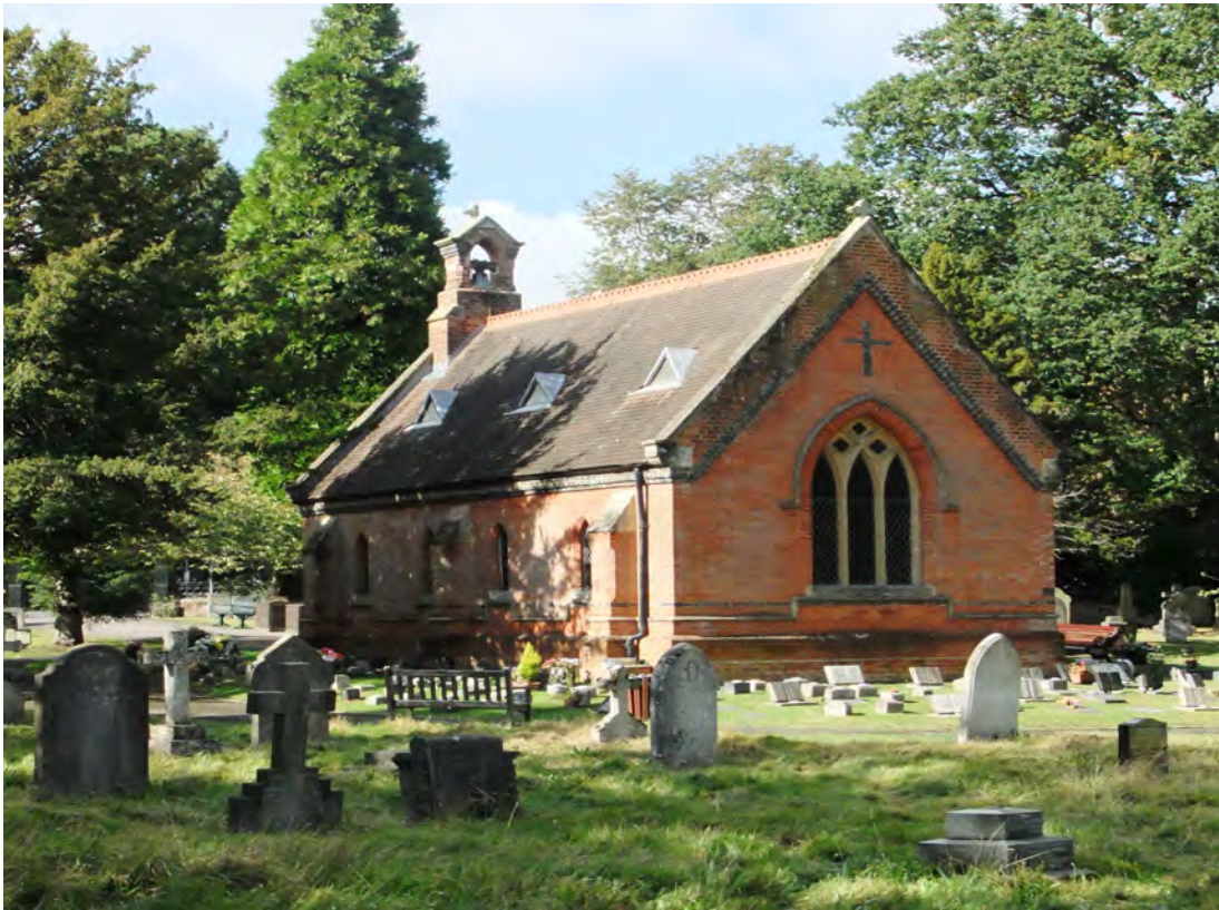
Illustration 13 The 19 th Century Larges Lane Cemetery Chapel, built of local bricks from the Thomas Lawrence Brickworks. Its “Living Churchyard” is wildlife friendly.
