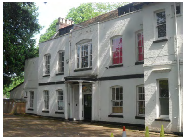
WR10: Old Bracknell House, Crowthorne Rd North
