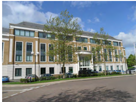
PW4: Arlington Square, off Downshire Way
