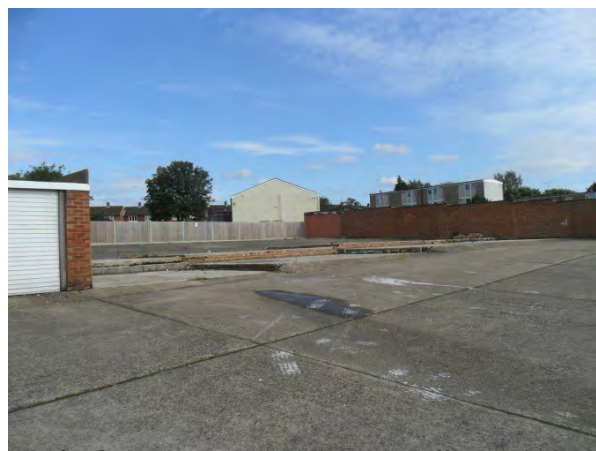
PW8: Clearance at garage block, off Merryhill Road
