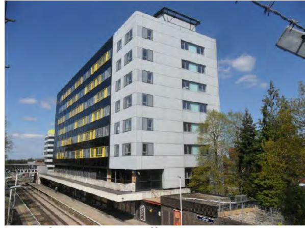
WR6: Station House: office to residential
