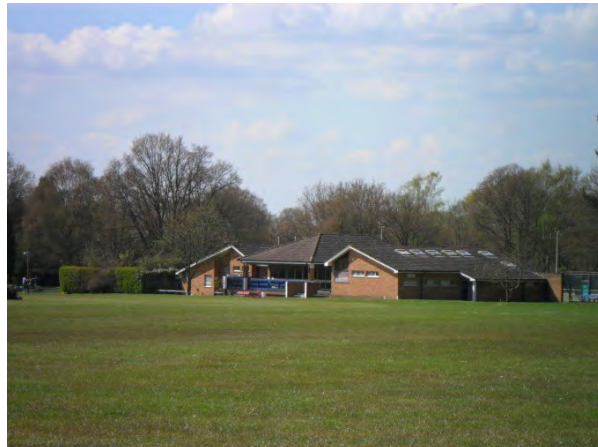
GH6: Great Hollands Recreation Ground Pavilion, South Road (being replaced in 2018)
