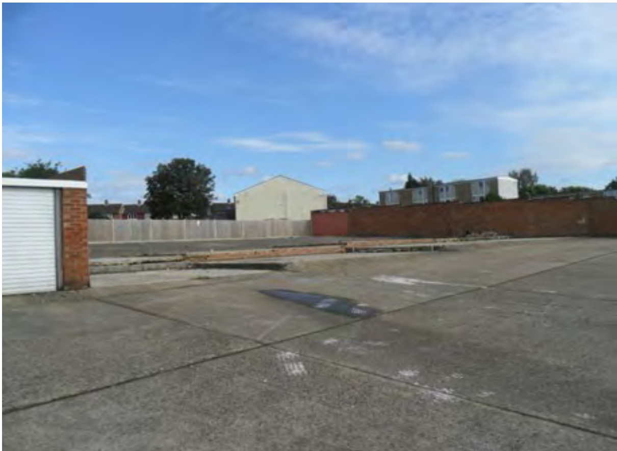
Illustration 9 Clearance at garage block, off Merryhill Road
