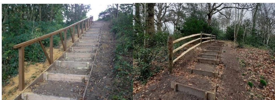
Newly refurbished steps at Longhill and Clintons Hill
