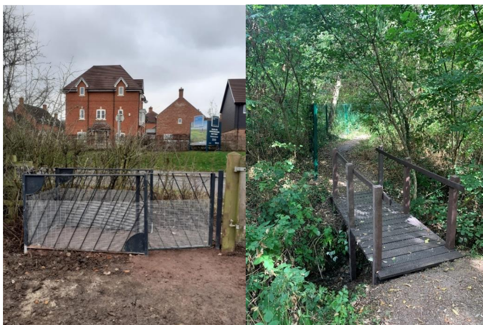
An example of the new bespoke gateways installed across the sites & new recycled plastic bridges within Piggy Wood
