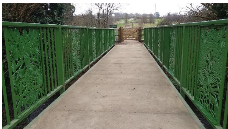
Bespoke bridge railings over the Cut river at one of the entrances to Larks Hill
