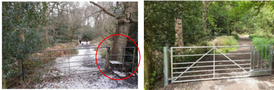
Figure 19 Step over stile (left) removed and replaced with kissing gate (right).
