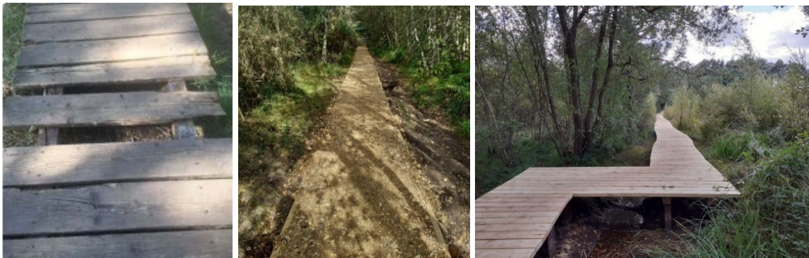
Figure 24 Before and after pictures of footpath/boardwalk improvements
