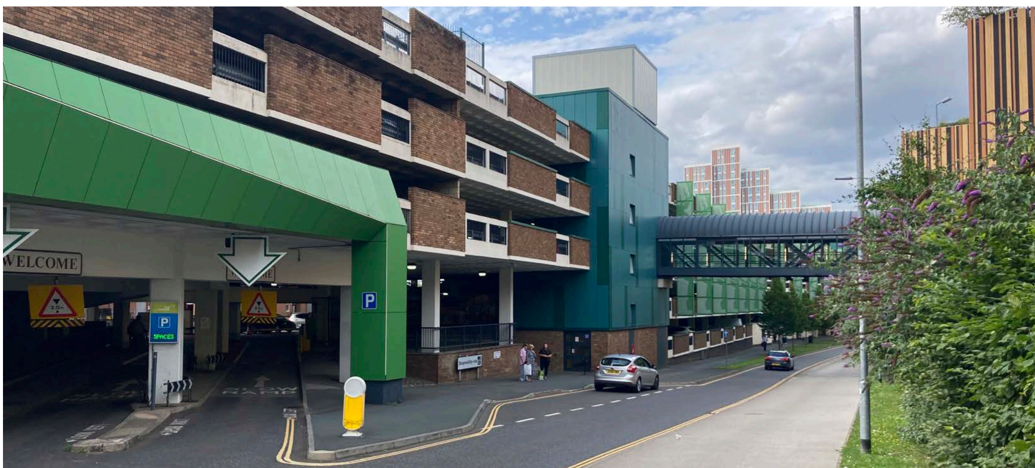
High Street Car Park – recently closed
