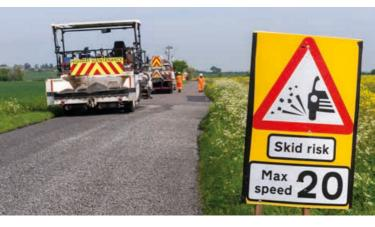
Within a week, we return to spray the new surface again to lock in any loose stones. Surface dressing seals the existing road surface, making it waterproof to prevent water from entering and weakening the structure. This helps to avoid cracks and potholes, protects against sunlight damage, and provides a new, hard-wearing surface.
