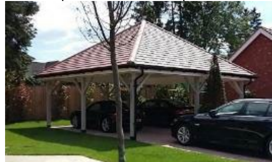
Figure A5 – An example of a well-designed and well-used carport in a new development
