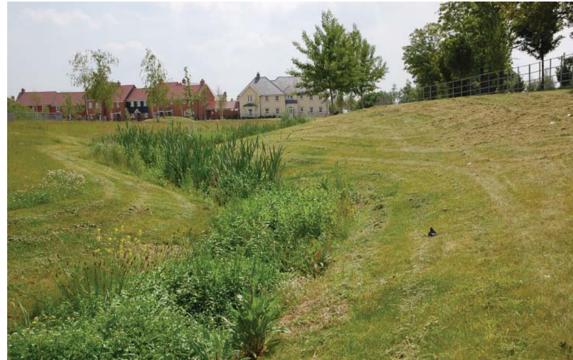
Example of SUDS that incorporate natural landscape and ecology as part of technical engineered drainage solutions
