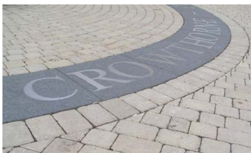
Photo 1 – Paving at Crowthorne Square
